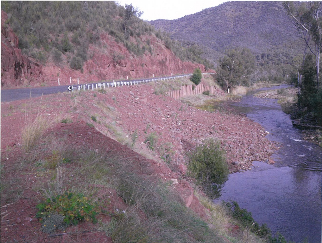
Figure 17 Repaired road wash-out on Macalister River
