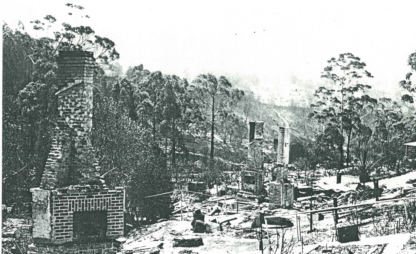
Damage to Tasmanian houses in the Hobart fire of 7 February 1967.
