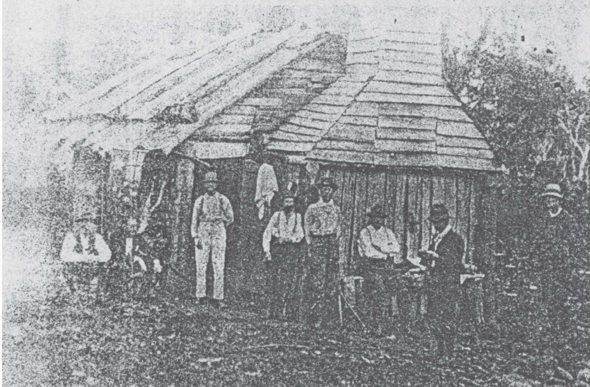
A large summer party at Miller's Hut.. Note the original bark roof with the substantial supporting log framework.
