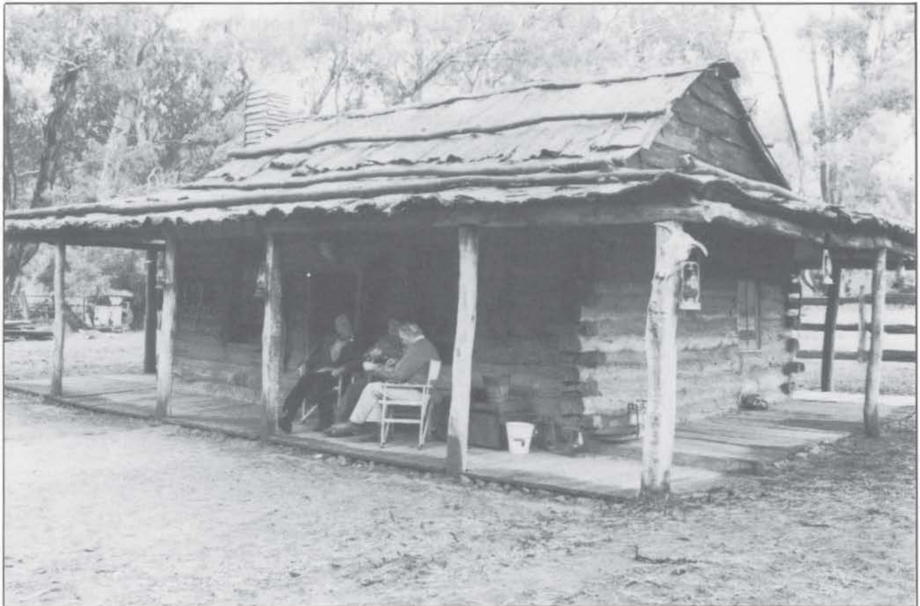
Harry Smith's hut fully restored to its original condition.
