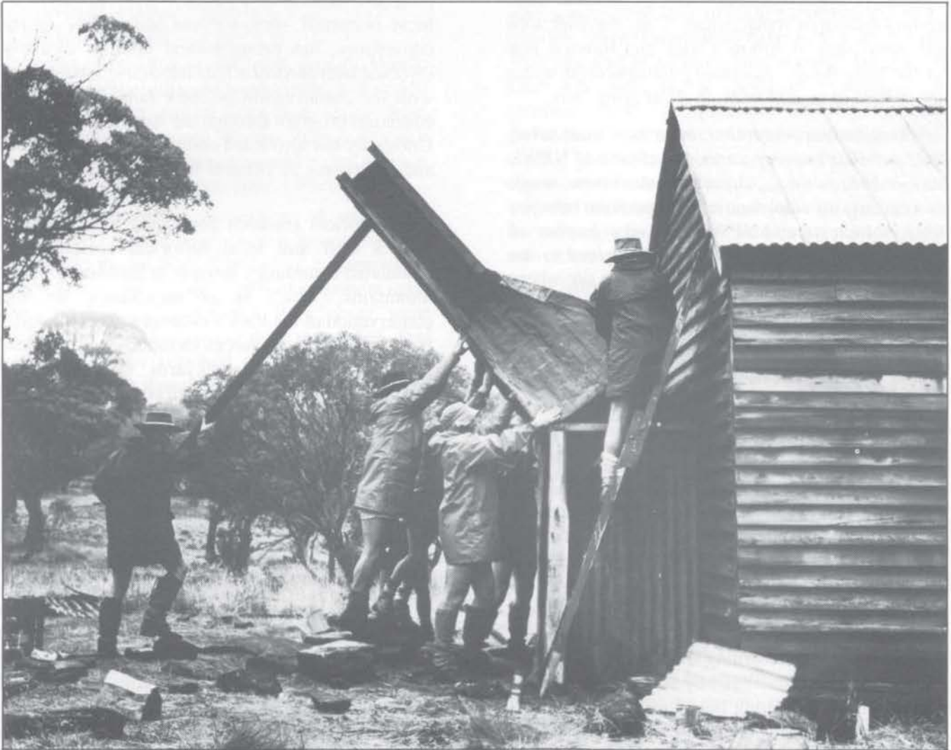
A new chimney for one of the Kosciusko huts courtesy of the Kosciusko Huts Association. (Dean Turner)
