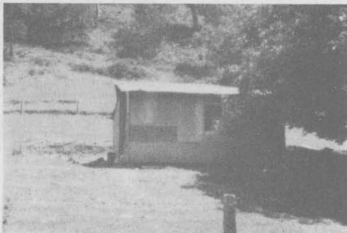
Beveridge hut - replacement of the original home burnt in January 1939 bushfires.
