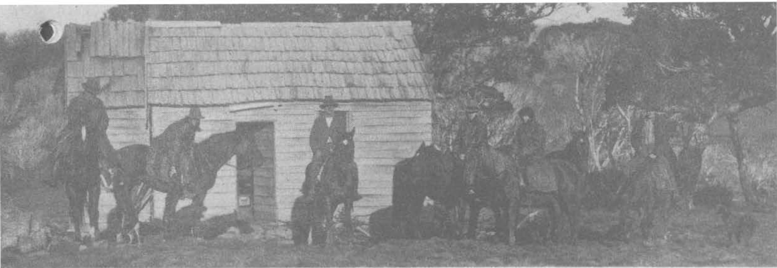
P. J. Kelly, Bill Batty, Geo. S. Fitzgerald, Andy Kelly, Keith Kelly and D'Arcy Fitzgerald (all but Andy Kelly since passed on) outside Fitzgerald's hut (pre 1928 - re-roofed with iron in 1929).
