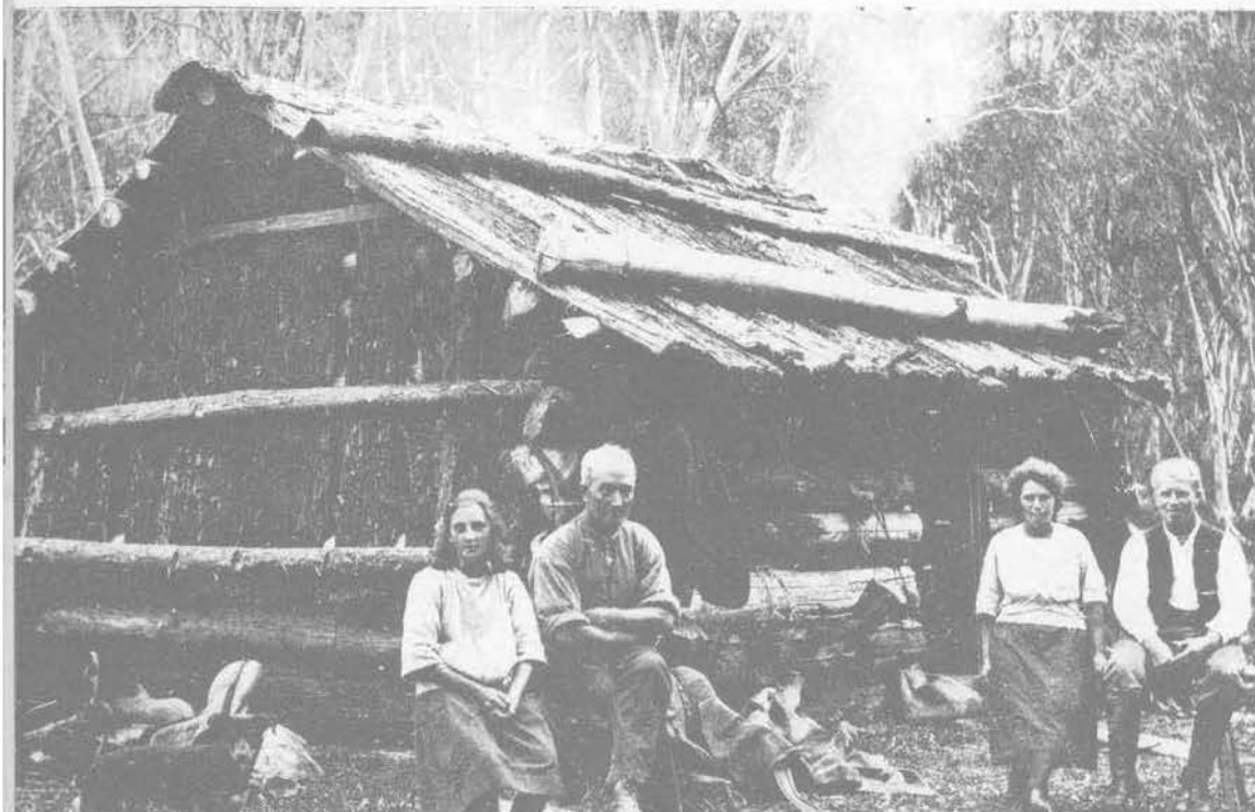
Blair's second hut, built in 1931 to replace No. 1 was of part horizontal log and part vertical bark construction with a bark roof, anchored by two substantial logs. There was no exterior chimney, but it featured an interior fireplace.
